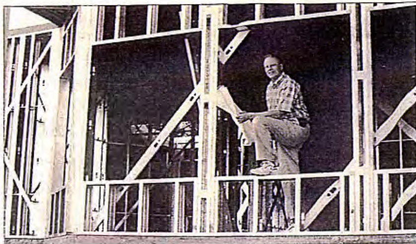
Martin McLeod supervises construction of his White Rock steel-frame house.
